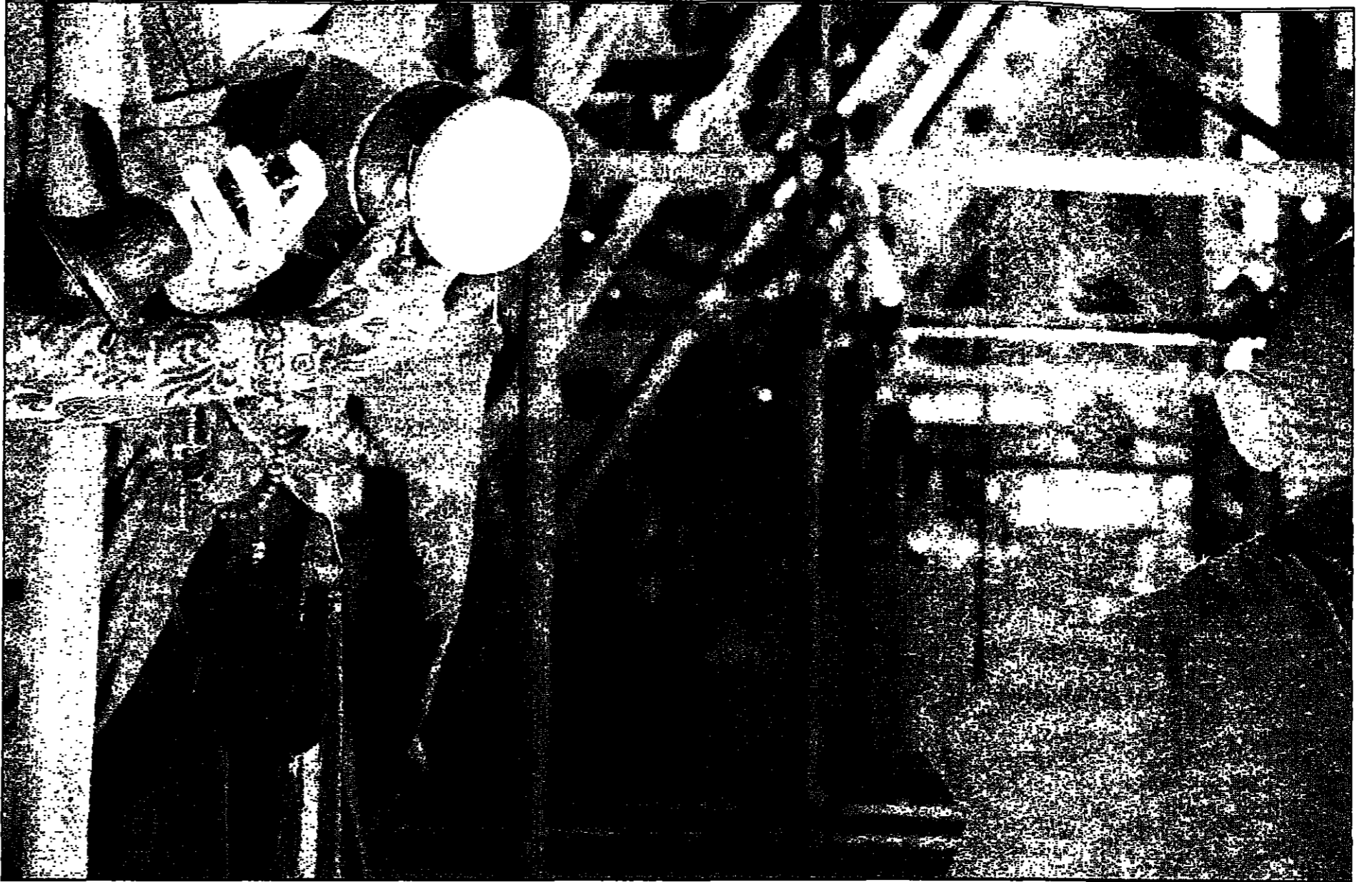
Meditation among the scaffolding... Buddhists yesterday at the Eskdalemuir temple where cracked beams threaten to make the roof unsafe
